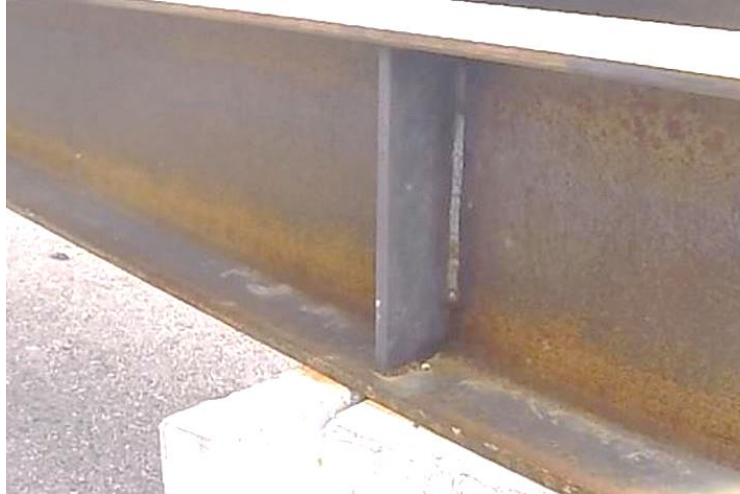
Figure 9. Visual Weld Inspection on the Small Bridge, E004
