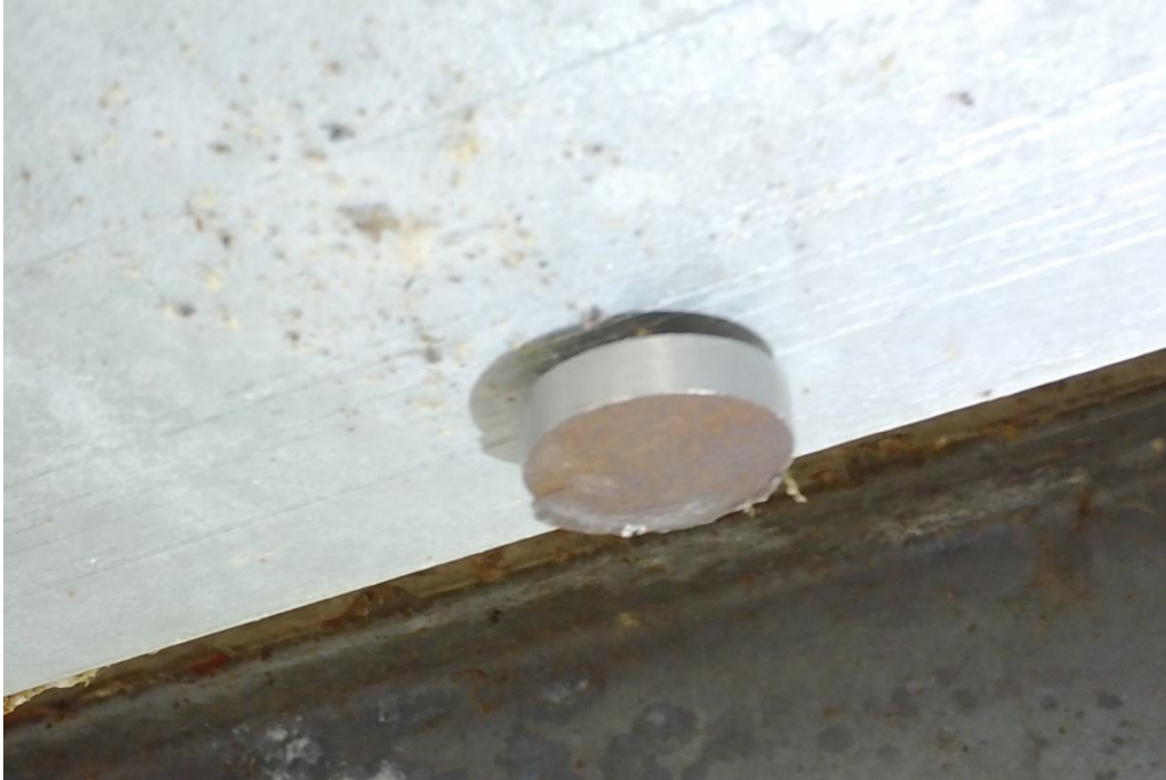
Figure 28. Photo of the Test-Piece Taken by DJI Mavic, UWRL Bridge, Bright Condition, Oblique Camera Angle, E012
