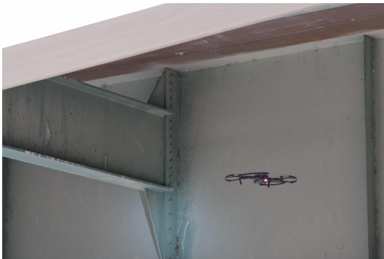
Figure 49. UAS Flying Under the Bridge.
