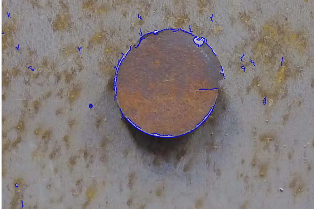
Figure 29. The Detected Crack Using Image Processing Techniques on the SMASH Lab Images (Laplacian of Gaussian), E014
