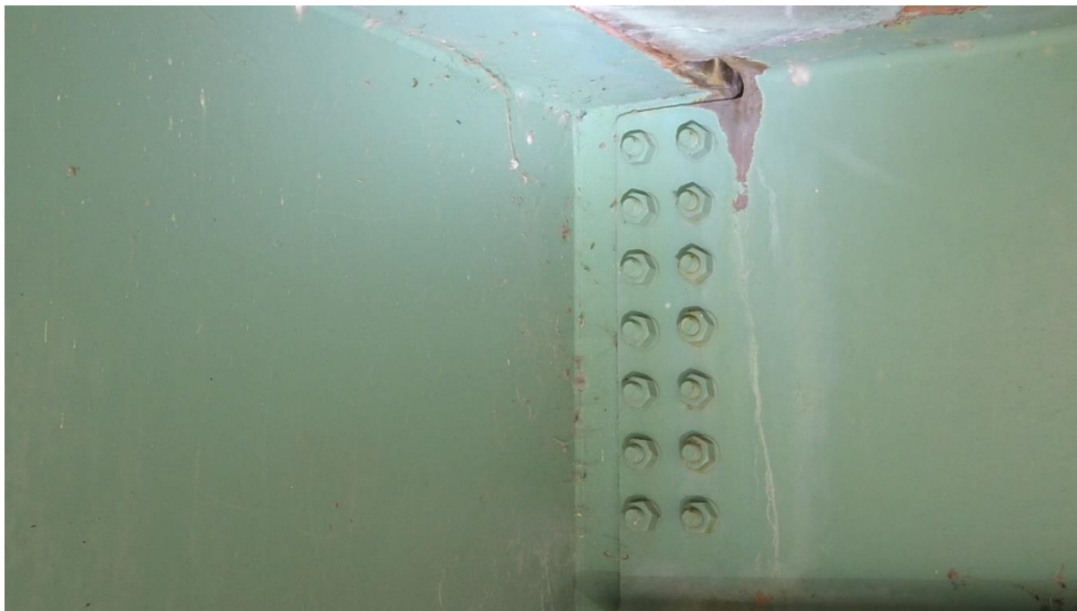
Figure 51. First Floor Beam on East, Northern Corner, No Noticeable Crack, E021
