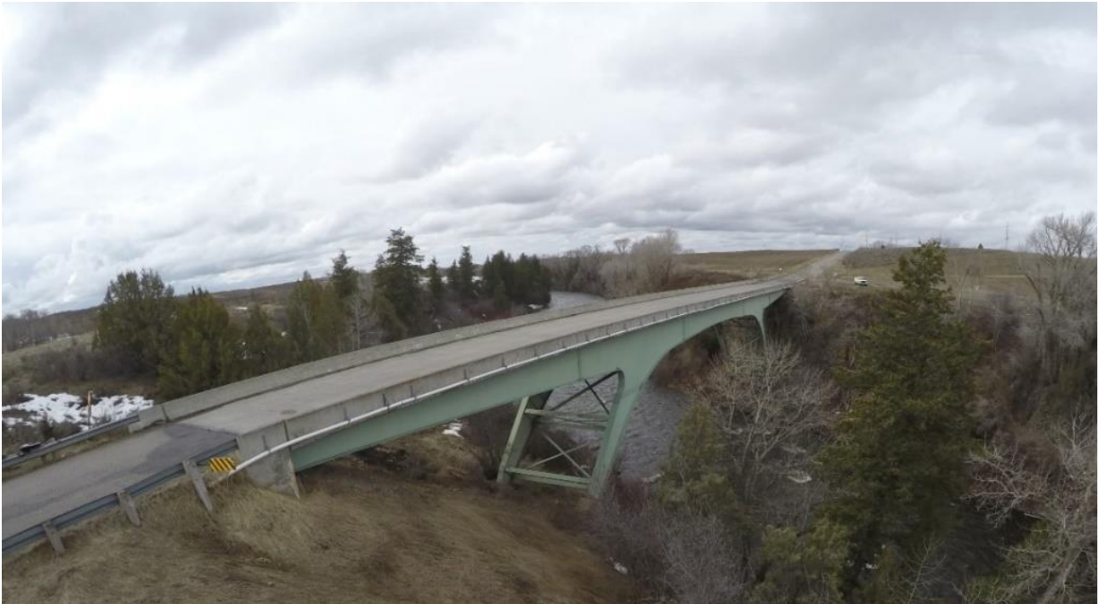
Figure 47. Northern Girder of the Fall River Bridge.
