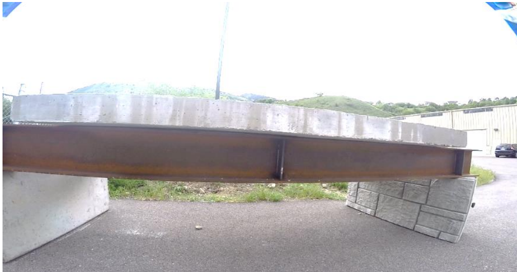
Figure 8. Steel Girder Surface Corrosion and Rust in the Image Acquired by UAS, E004
