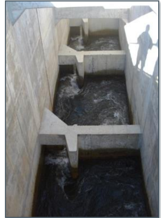
VSF at Coimbra dam
