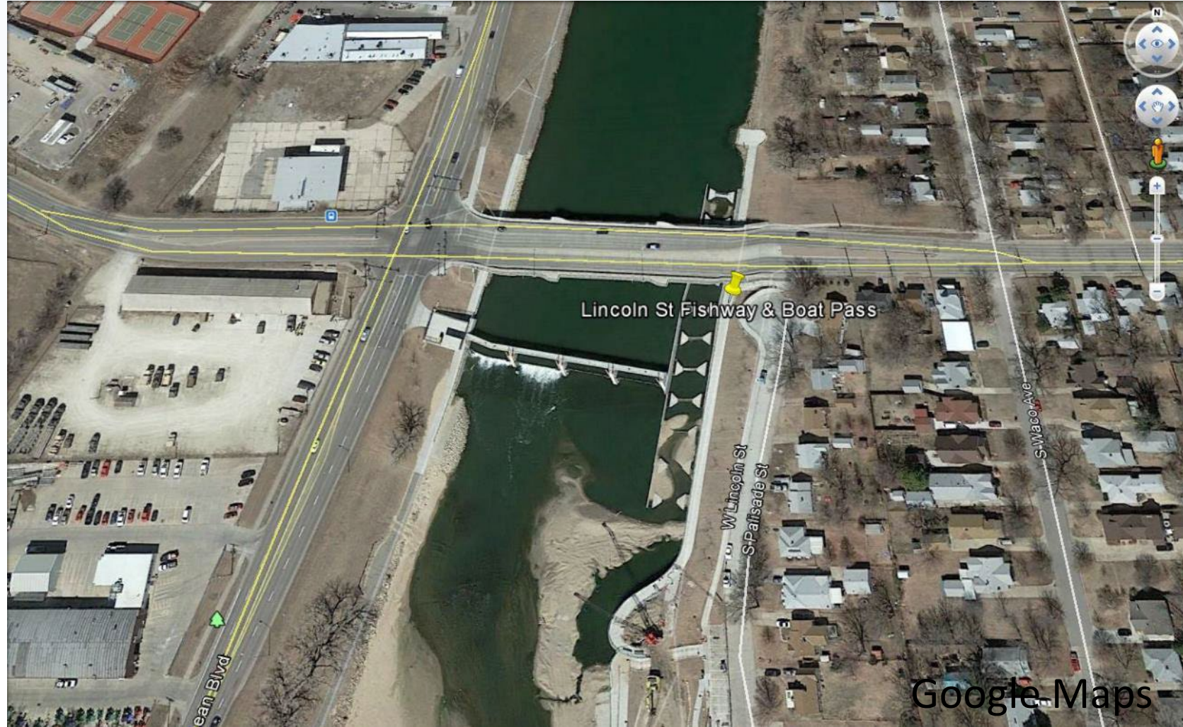
Lincoln Street Fishway, Wichita, Kansas
