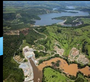
Amador Aguiar I Dam
