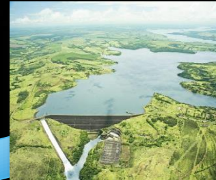
Nova Ponte Dam
