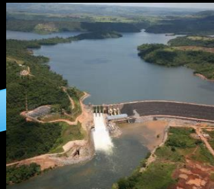
Amador Aguiar II Dam
