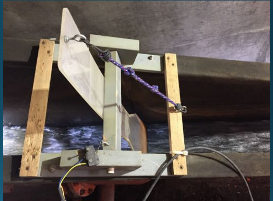
Black River Pump Station WA. Fish counter
