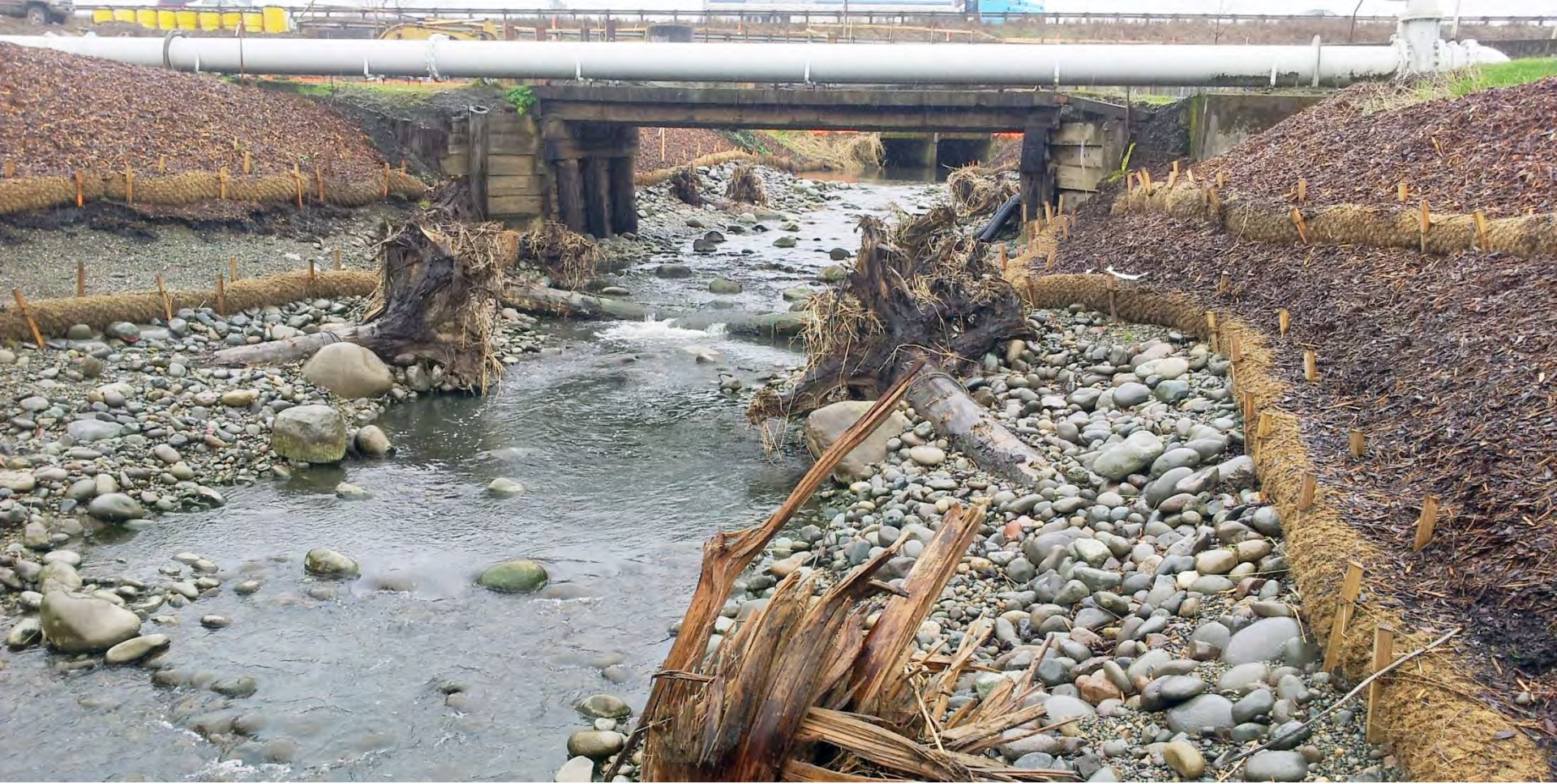
China Creek – Completed Project
