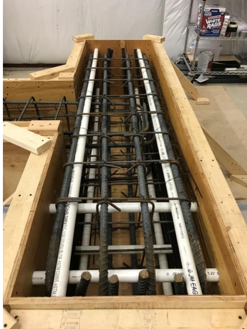
Figure 4.5: PVC tubes passed through the exterior column cages
