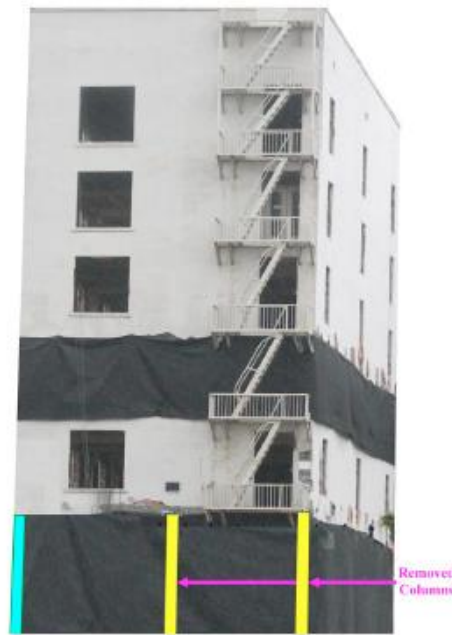
Figure 2.5: Six-story building tested by Sasani and Sagirolu (2008)
