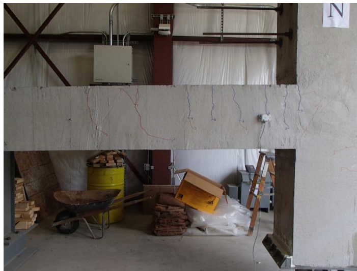
Figure 5.40: Cracks near the north column (Specimen 3)
