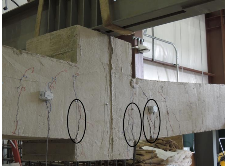
Figure 5.20: Critical flexural cracks near the center column (Specimen 2)
