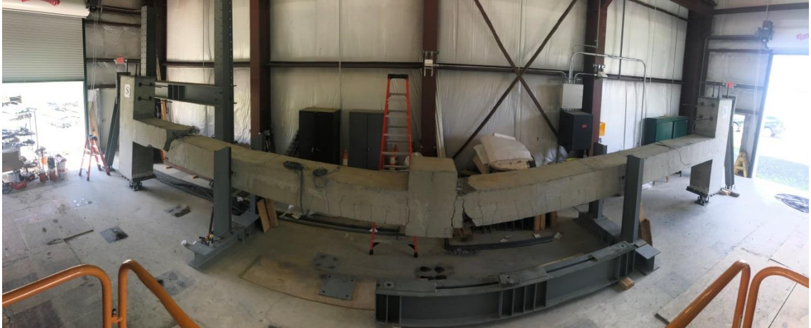
Figure 5.42: Specimen 3 condition at the end of the test
