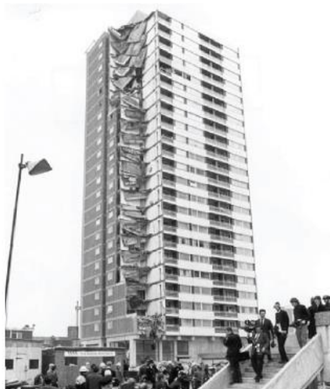
Figure 1.2: Partial collapse of the Ronan Point apartment building (Pearson & Delatte 2005)
