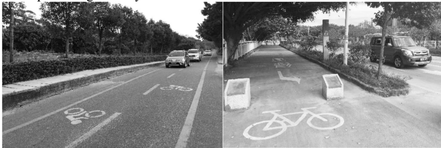
2B in-roadway bike lanes
