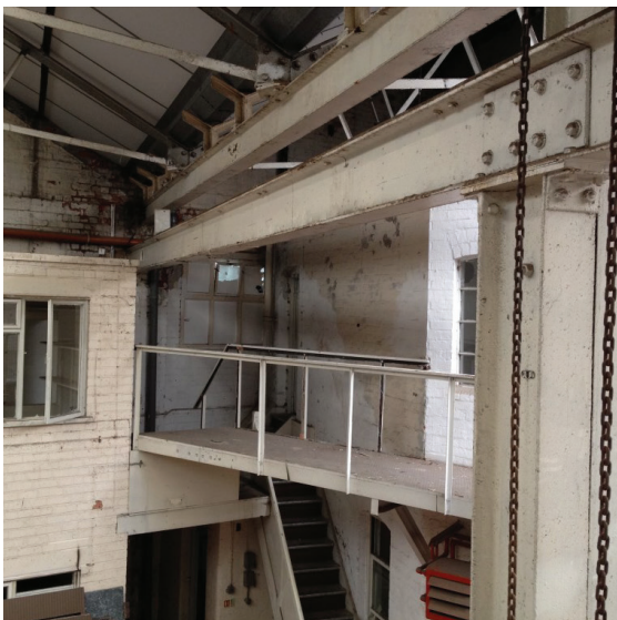
Figure 8: Before Renovation - Catwalks
