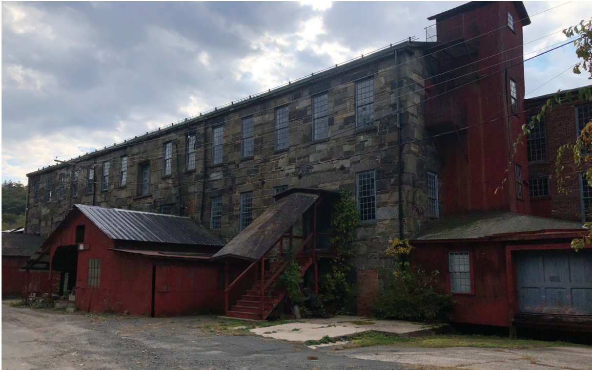
Figure 44: Building Six Existing Front Facade
