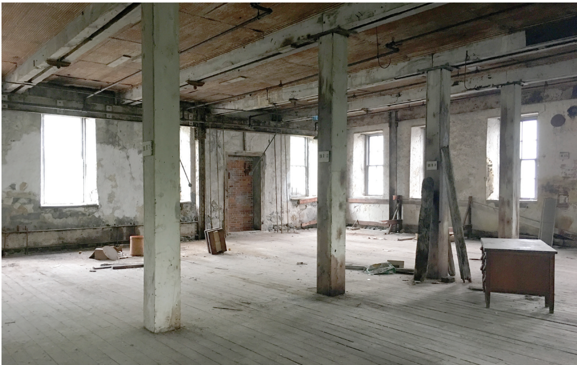
Figure 45: Existing Interior of Building Six, June 2016
