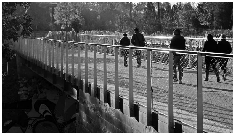
Figure 4. Eastside Trail Bridge with Elberton Granite and Stainless Steel Railing
