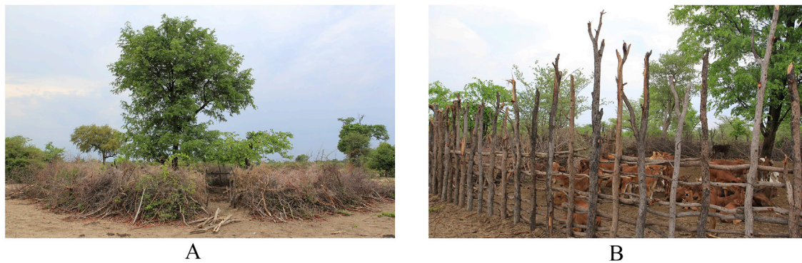
Fig. 2. Traditional kraal structures in northern Botswana. A: thorn branch style construction, B: thick wooden branch construction. Photos by E. LeFlore.
