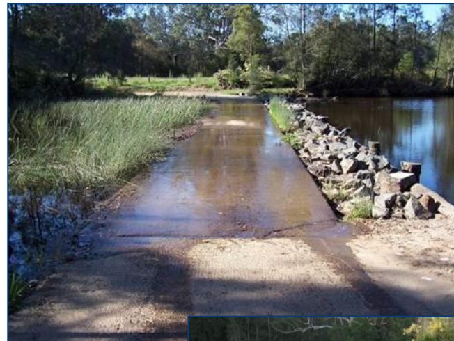
Culvert and partial-width rock ramp fishway
