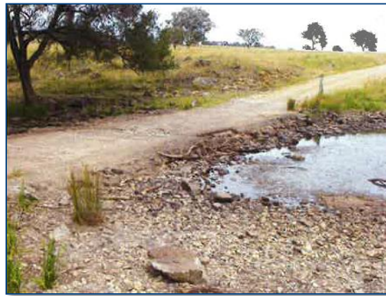
Causeway with narrow pipe restriction, now with box culvert
