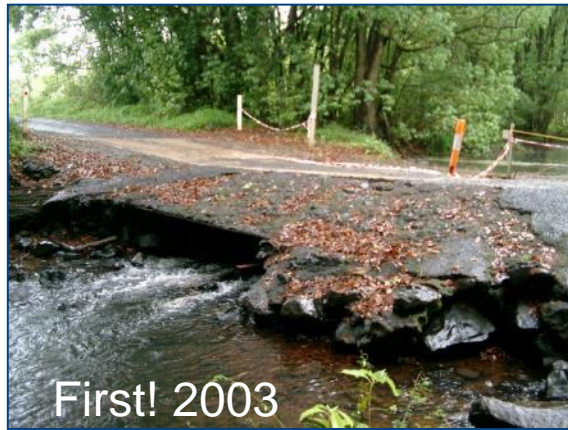
Causeway with narrow pipe restriction, now with bridge
