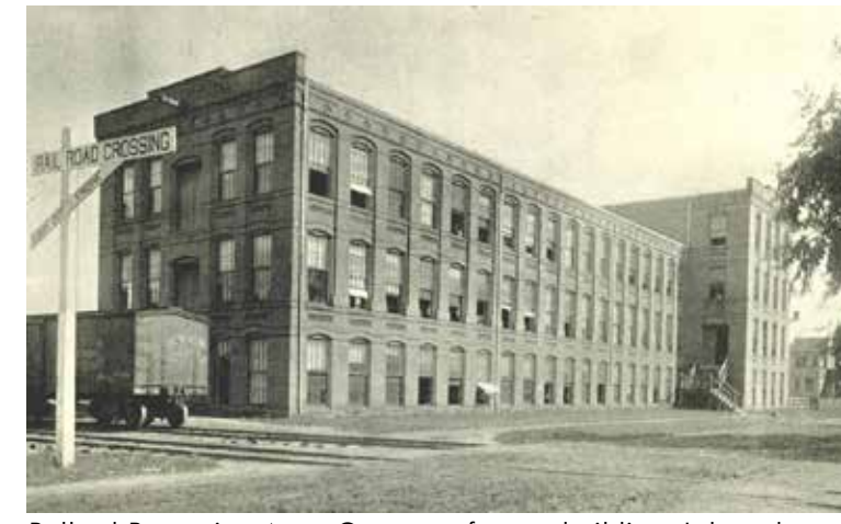
Bullard Repeating Arms Company factory building. It later housed the Indian Motorcycle Factory. 1892
