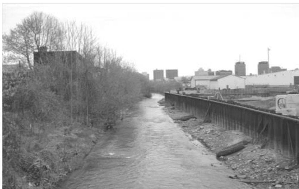
Figure 1: Channelization of Onondaga Creek Syracuse, NY. Source: Photo by R Smardon
