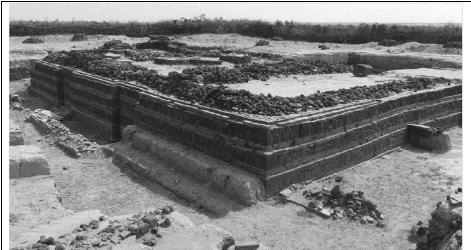
Figure 8 Graduated Masonry at Adulis Temple A
