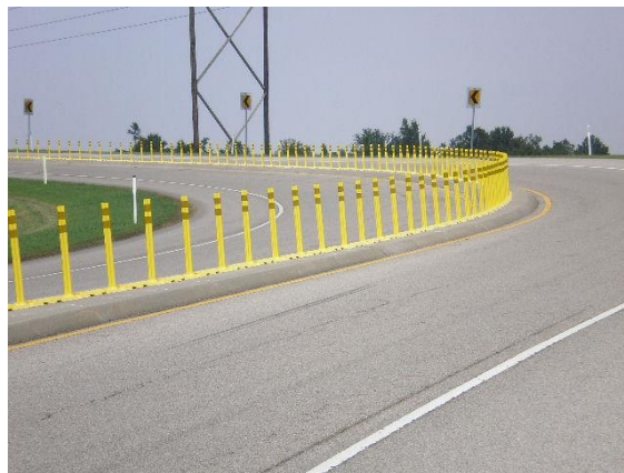
Figure 3 - Post Mounted Delineator
