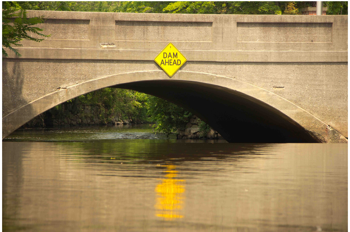
Figure B.1. Some dams in Massachusetts feature warning signs to alert those upstream of the dangers ahead. Many do not, however.
