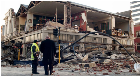
a) Damage caused by the earthquake on 4 September 2010 in Christchurch, New Zealand (Photo: www.foxnews.com )
