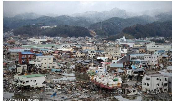
b) Damage caused by the tsunami on 11 March 2011 in Kesenuma, Japan (Photo: http://www.dailymail.co.uk )
