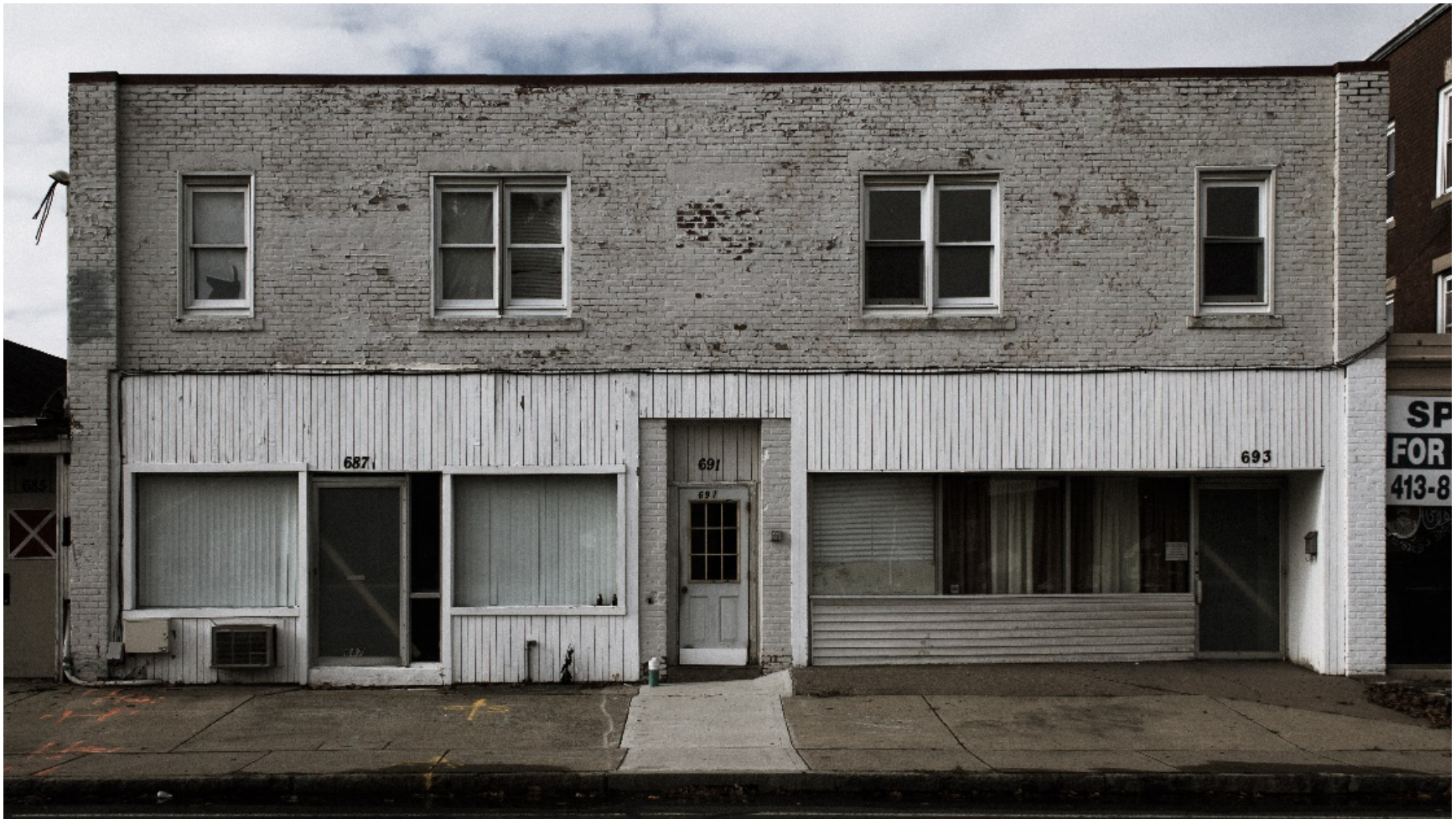
Figure 119: 687 – 693 Grattan Street - Vacant building across from Aldenville Commons, next to TD's Pub and former bowling alley
