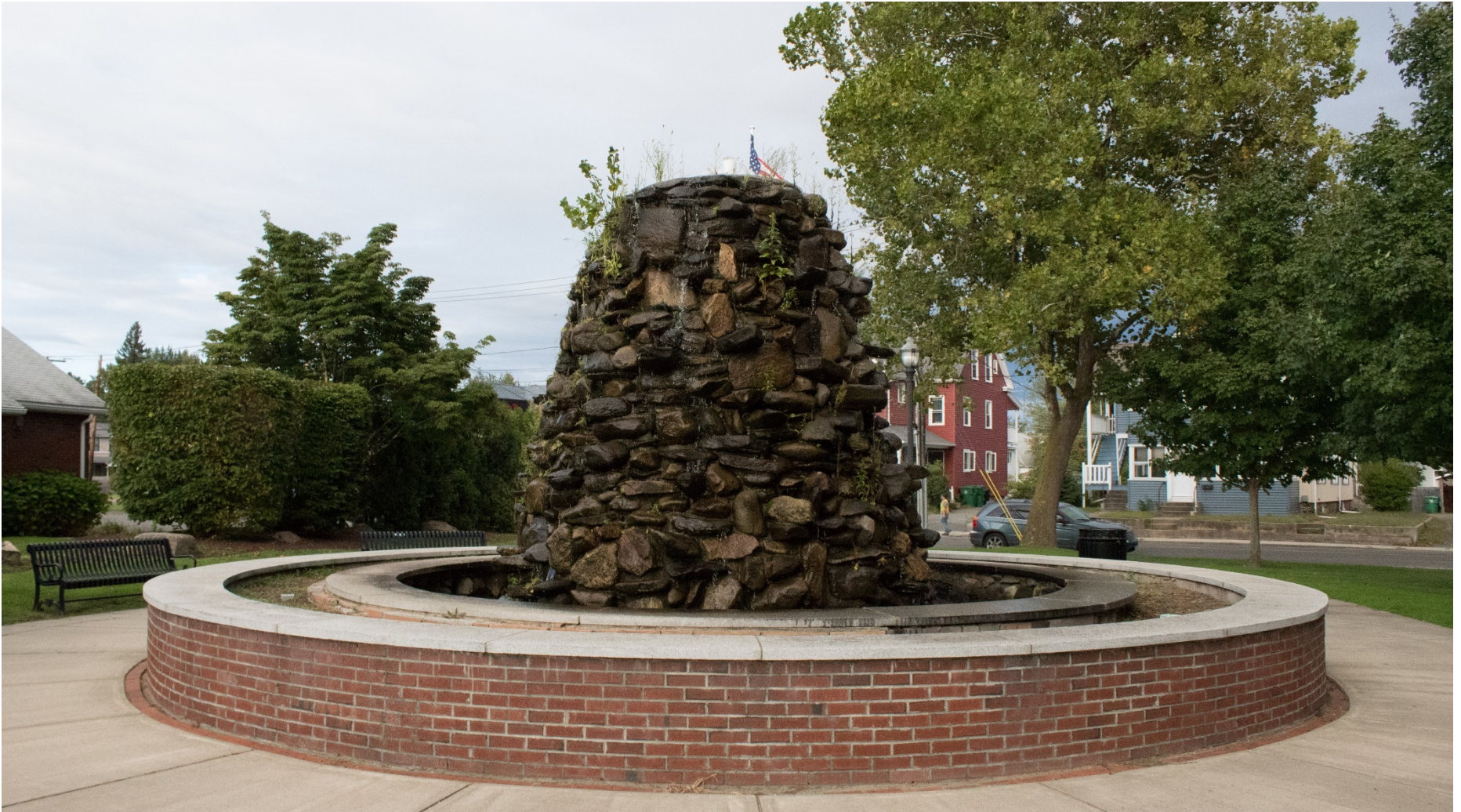
Figure 112: Waterfall fountain at Aldenville Commons
