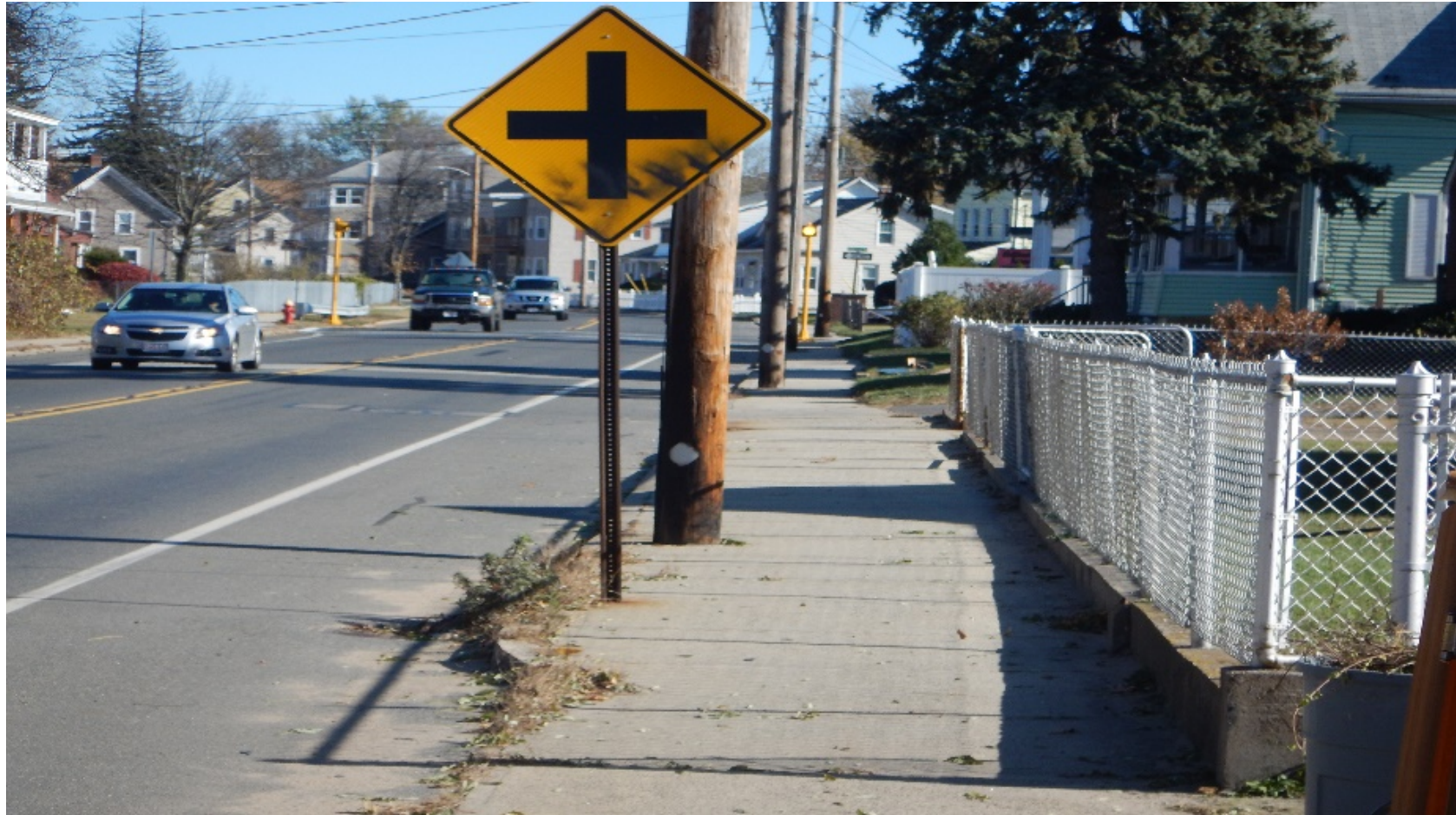
Figure 134: Existing conditions along McKinstry Avenue
