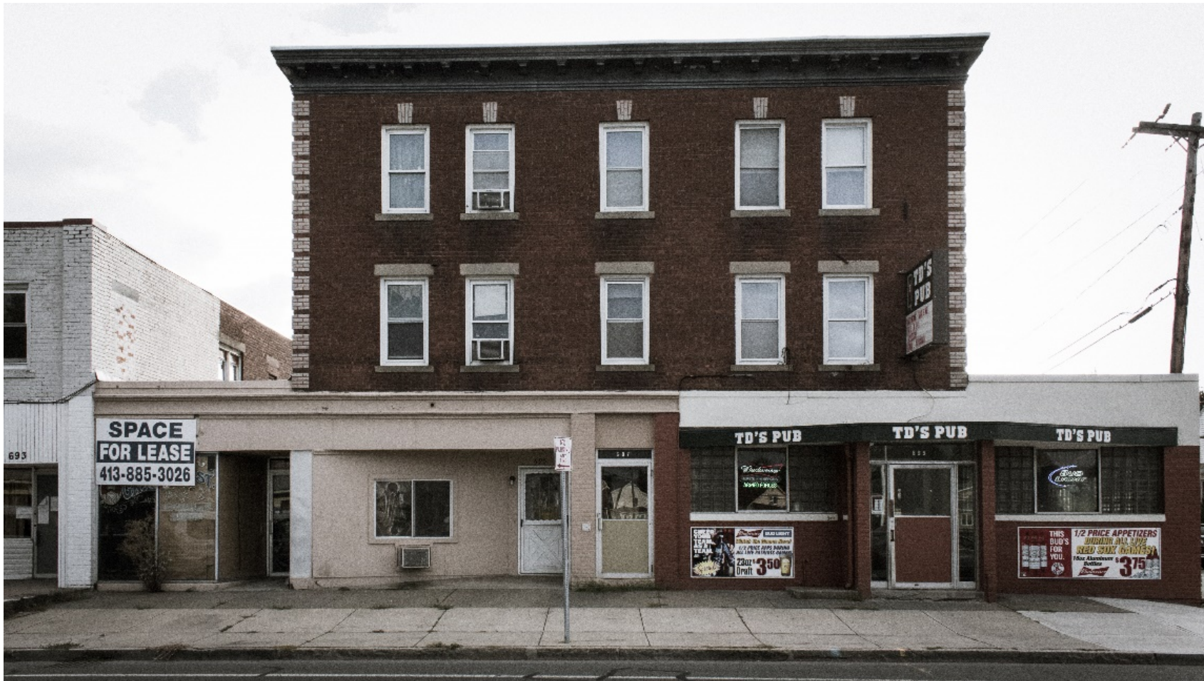
Figure 120: The Hammersleys Building
