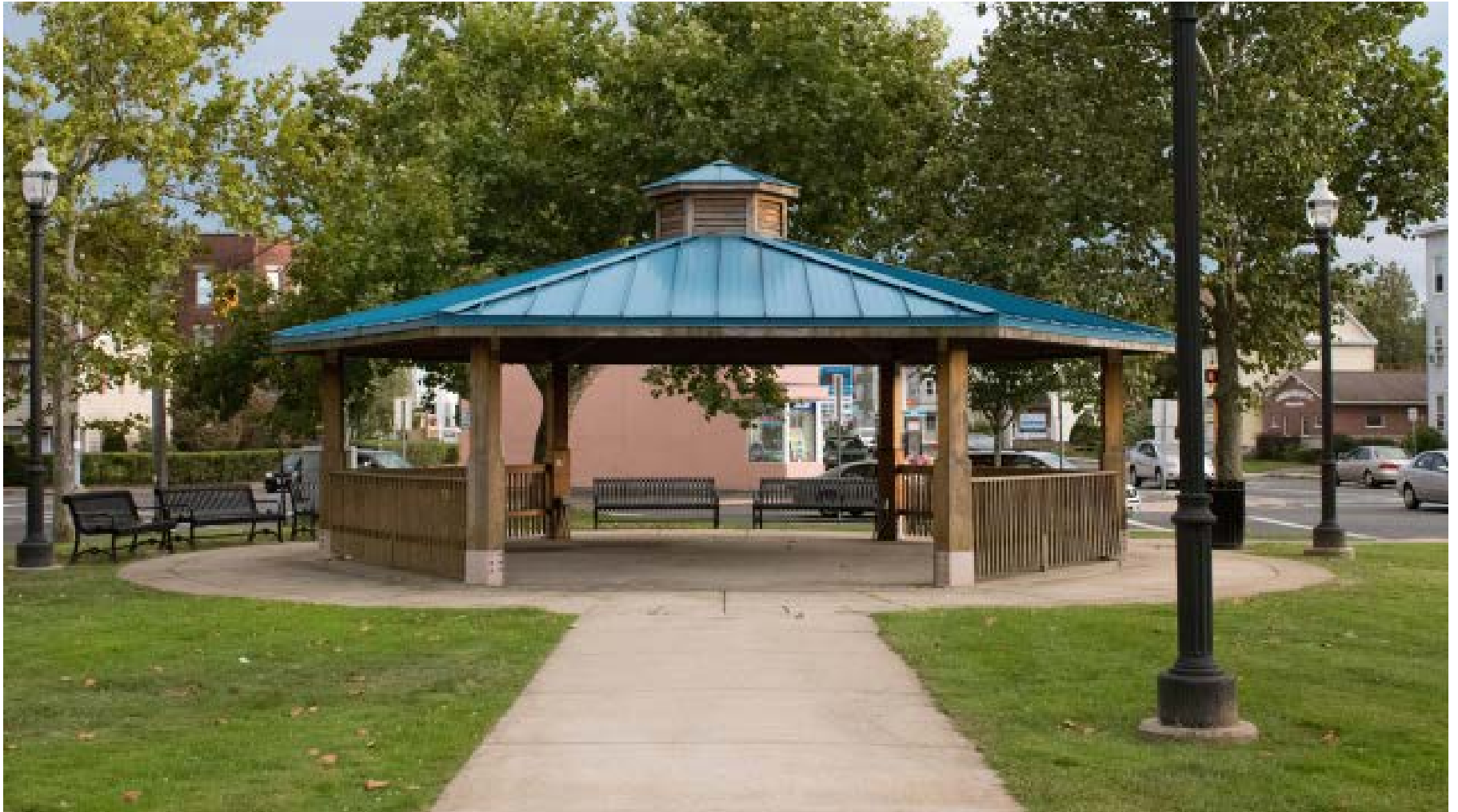
Figure 111: The Aldenville Commons gazebo viewed from the north
