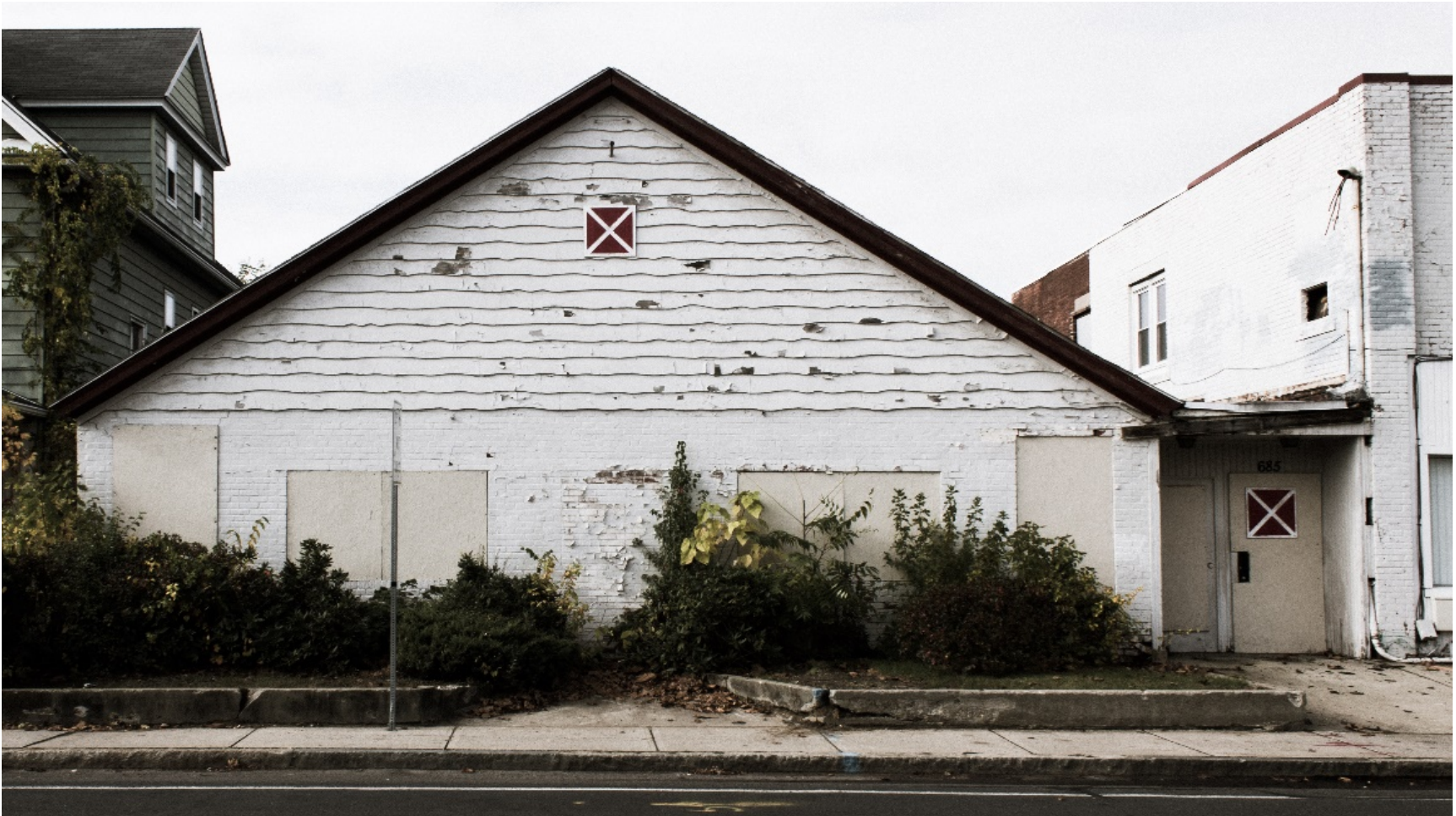
Figure 118: 685 Grattan Street - A former bowling alley
