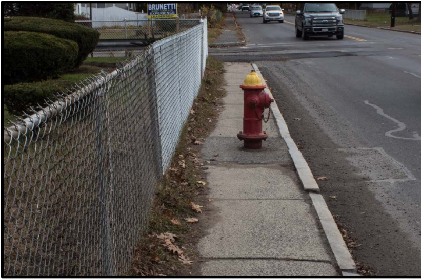
Figure 56: Fire hydrant obstructs sidewalk on McKinstry Avenue
