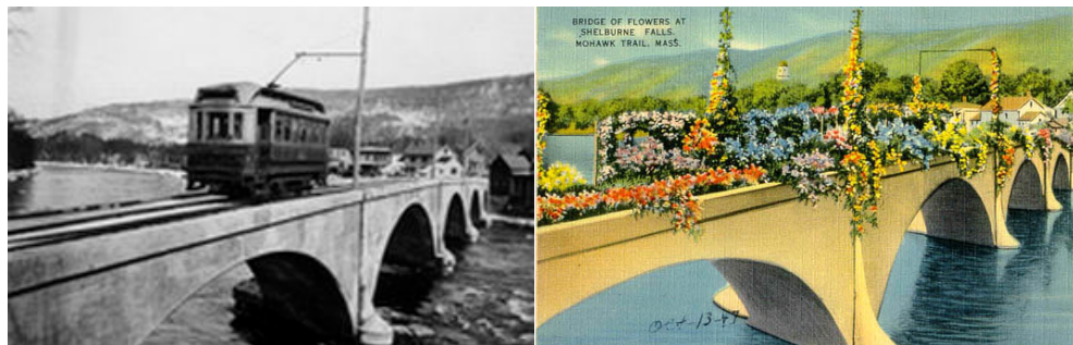
Figure 3.4 Bridge of Flowers Before and After Repurposing 41
