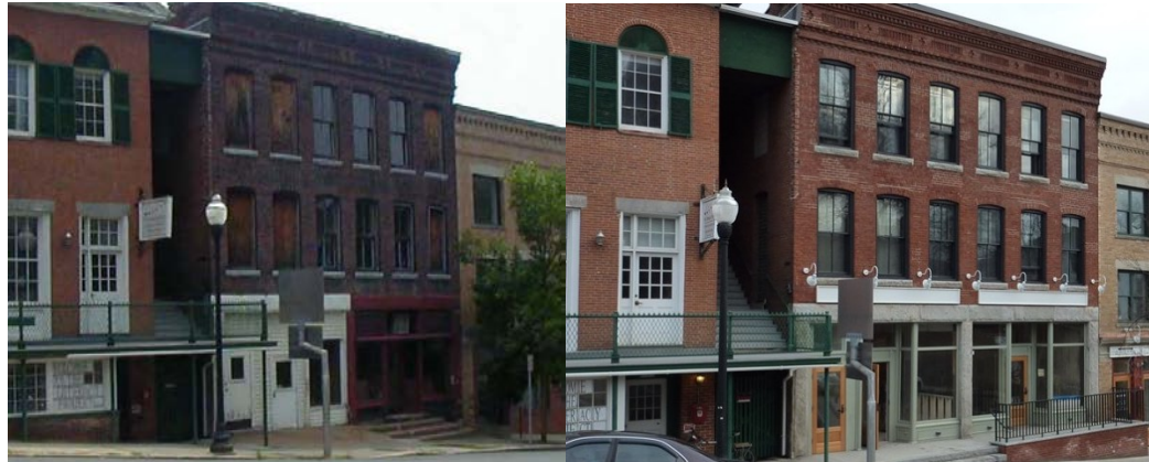
Figure 3.5: One Downtown Greenfield Property Before and After Renovation 45
