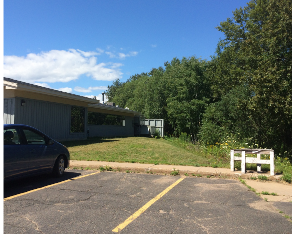
Figure 8. North side of the building, next to the Whetstone Brook
