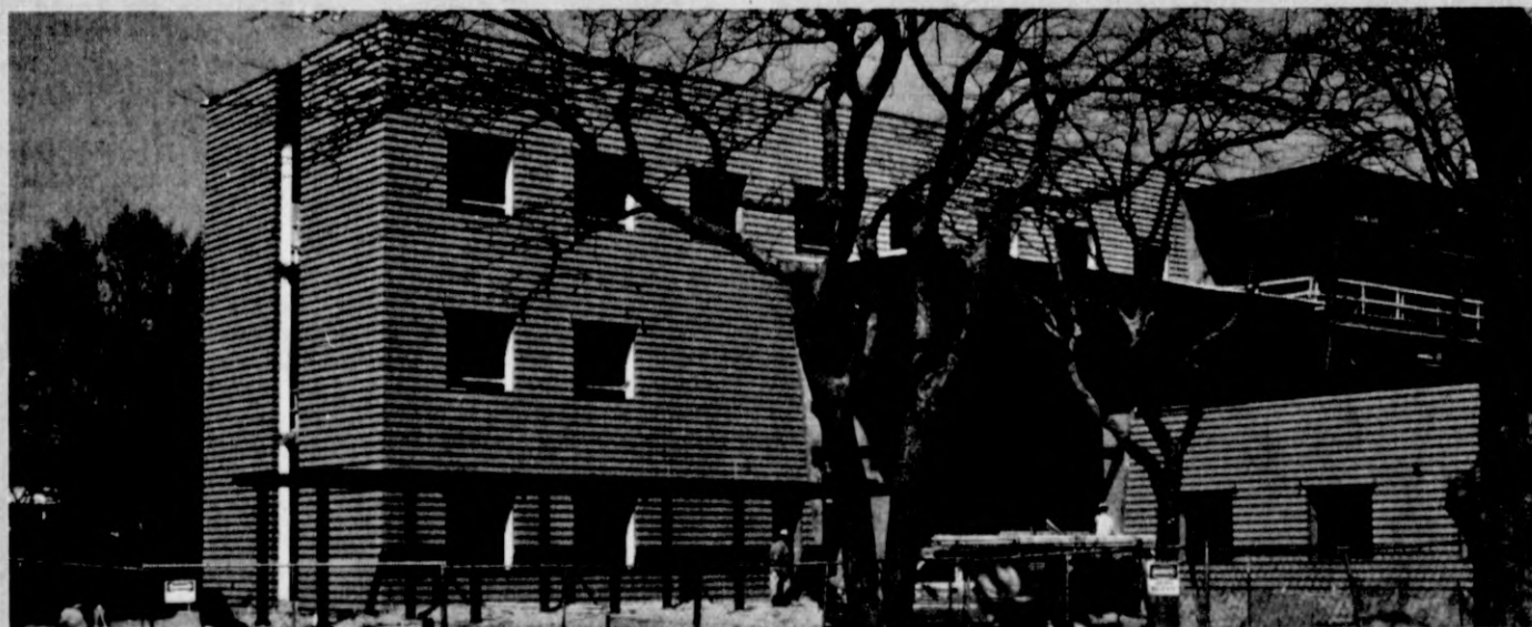
Still working: Lake Ontario Hall, GVSU's newest building, will be complete by the fall semester. Among the things it will house include 85 faculty offices, a Macintosh computer lab and student study areas. Construction began in September.
