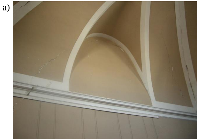
Figure 14. Cracks and local failure of the gypsum and timber ceiling. First floor, room on piazza Verdi
