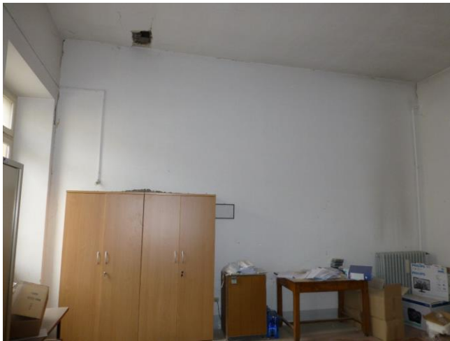
Figure 14. Cracks and local failure of the gypsum and timber ceiling. First floor, room on piazza Verdi
