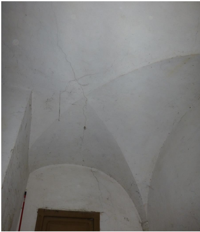
Figure 10. Widespread cracks having width smaller than 3 mm on a cross vault between ground floor and first floor. Shop on piazza Verdi
