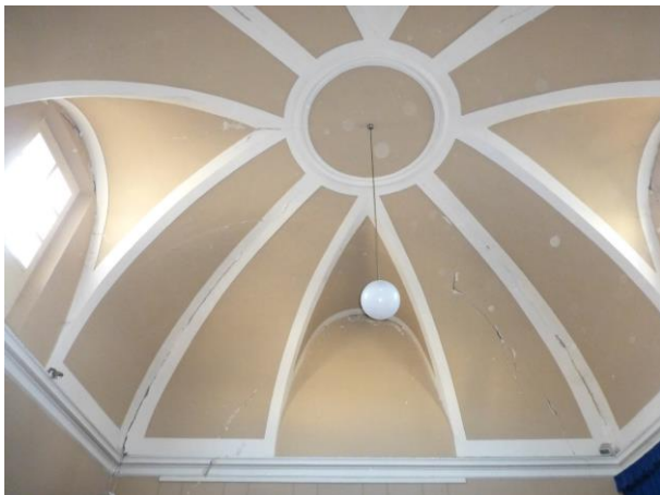
Figure 15. a) After August 24 th ; b) After October 30 th . Cumulative damage is evident in the lune and in the right adjacent web
