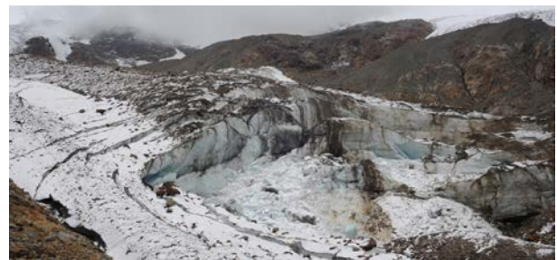
Figure 1. A large collapse occurred on the terminus of Forni Glacier in the end of Summer 2017.
