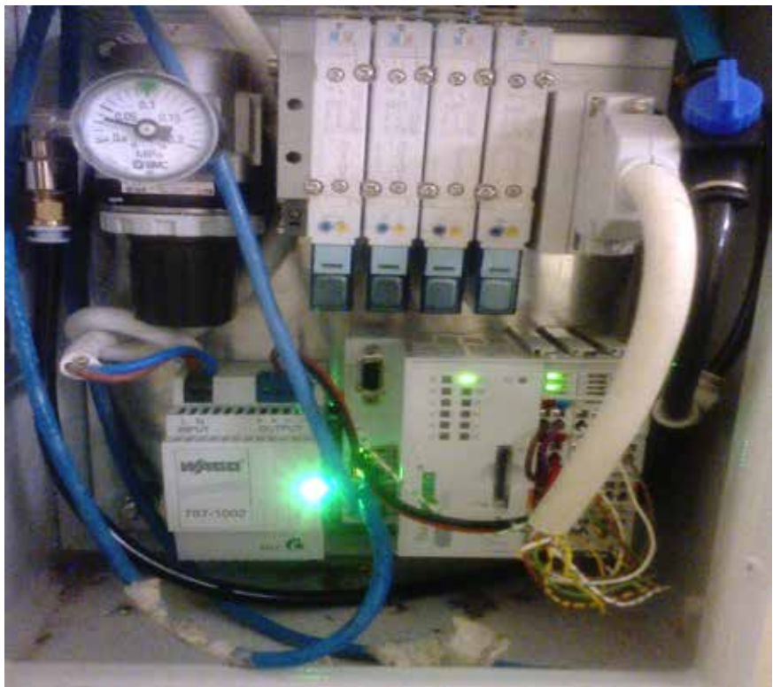
Plate 20. Filters (top) and programmable logic control (down) for SETIS™ type TIBs.
