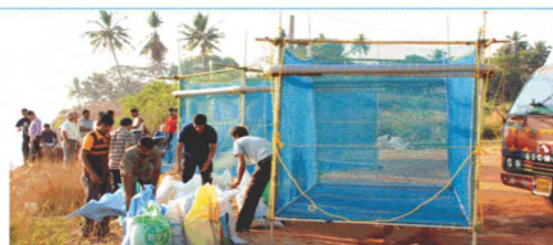
Fig. 9a. Illustration of Cage mooring with sand bags.
