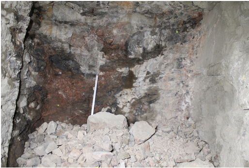
Figure 8.17: Photograph of the test location in tunnel wall test.
