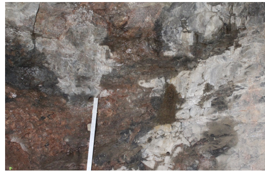
Figure 8.18: Photograph of the scanned area in tunnel wall test.
