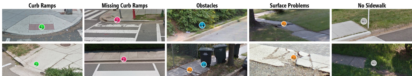
Figure 3: Project Sidewalk has five primary color-coded label types: curb ramps, missing curb ramps, obstacles, surface problems, and no sidewalk. The images above are example accessibility issues found by users in our public deployment.
