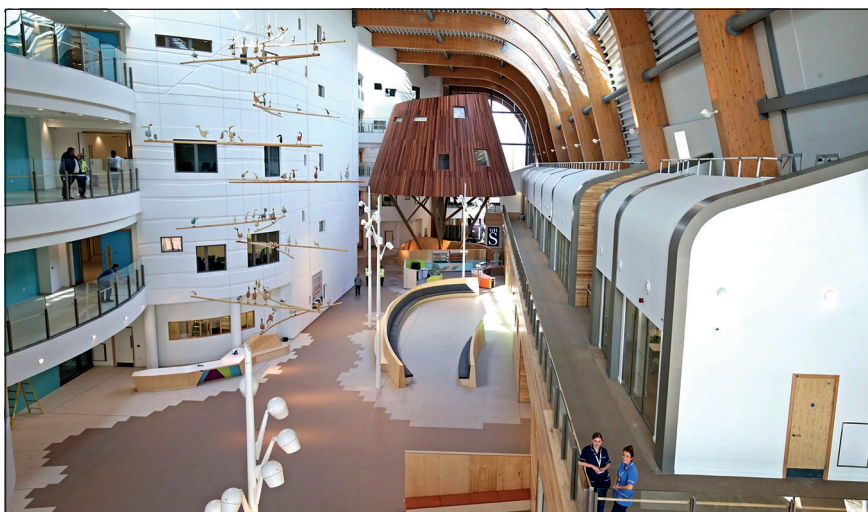
Figure 2. BIM enabled rapid delivery of Alder Hey Children's Hospital in Liverpool
