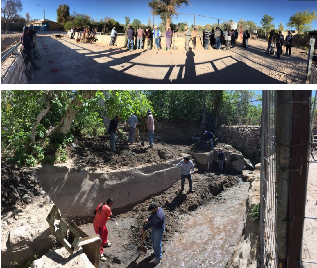
Figure 5.19 | Cleaning of the canals in Toconao
