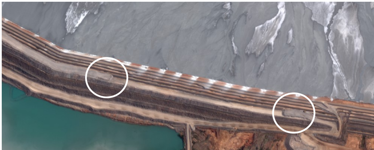
Figure 8 WorldView-2 imagery acquired at 10.28 am local time on 9 March 2018. White circles indicate construction activity, © DigitalGlobe 2018
