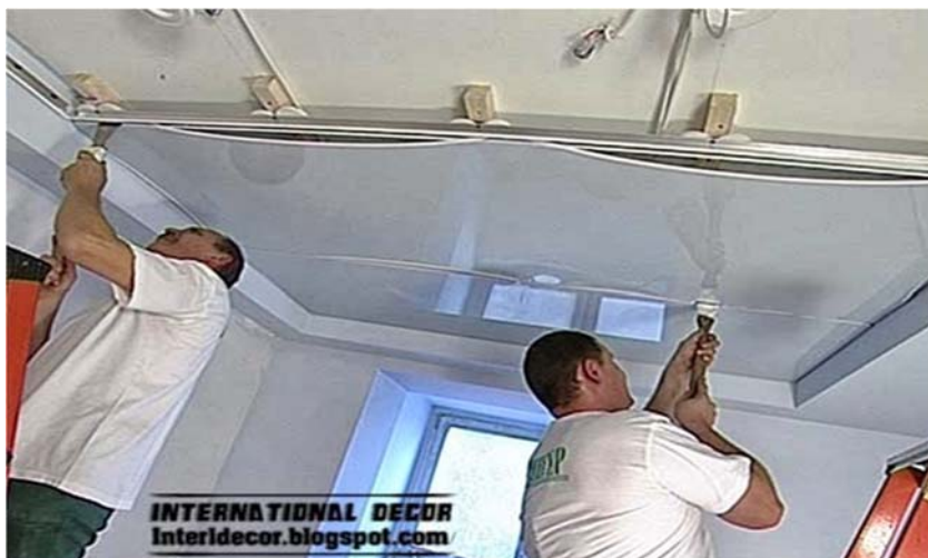
Figure 5: PVC stretched ceiling ideas, Source: [15]
