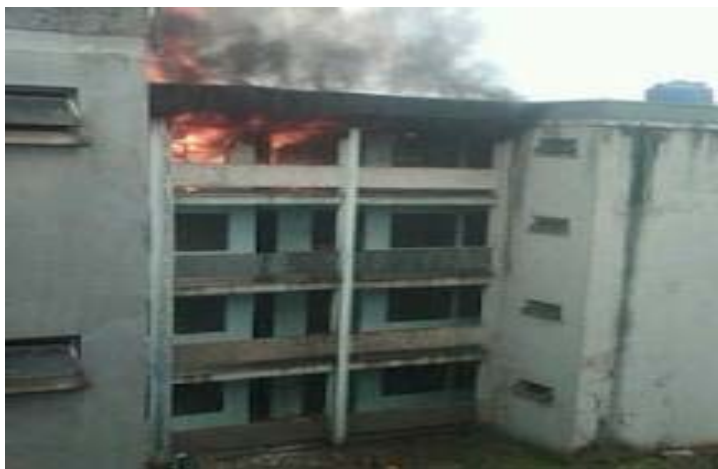
Figure 9: Early morning fire in the University of Lagos Hall of Residence Source:[36]
