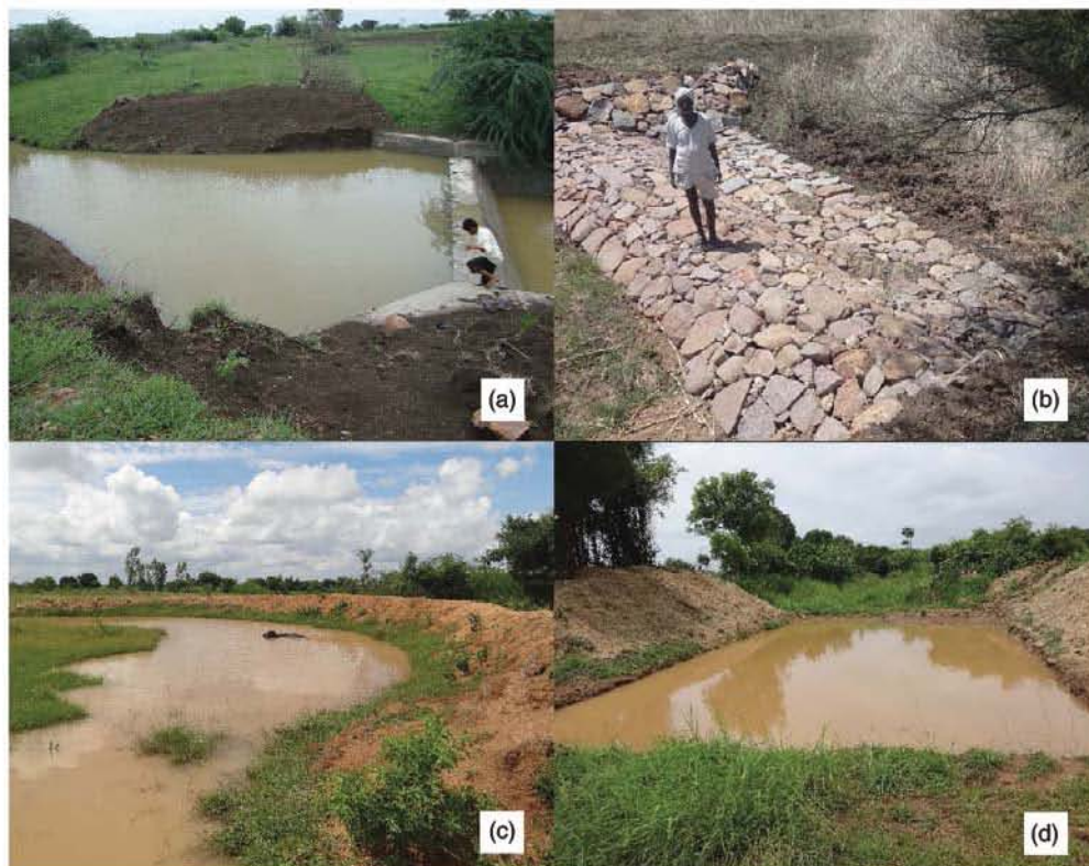
Fig. 5.3. Water-harvesting structures constructed in project villages: (a) check-dam in Shivampet; (b) rock-fill dam in Fasalvadi; (c) percolation tank in Chowtakur; (d) sunken pond in Sultanpur.
