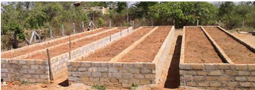
Fig. 9.2 Specially constructed root structures to assess genetic variability in root traits in large number of accessions. Note: Each of these structures measure 60-ft long, 5-ft tall and 10-ft wide and is constructed using cement bricks. A wall is built in the center for dividing the structures into two halves of 5-ft wide each
