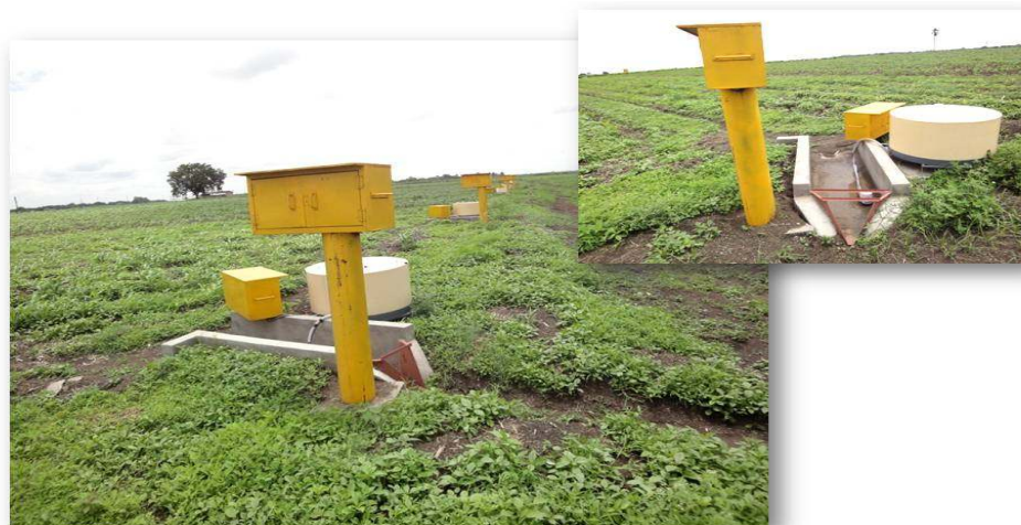
Fig. 2. A field view of the installed integrated digital runoff and soil loss monitoring unit (IDRSMU), photo in insert is close up of IDRSMU
