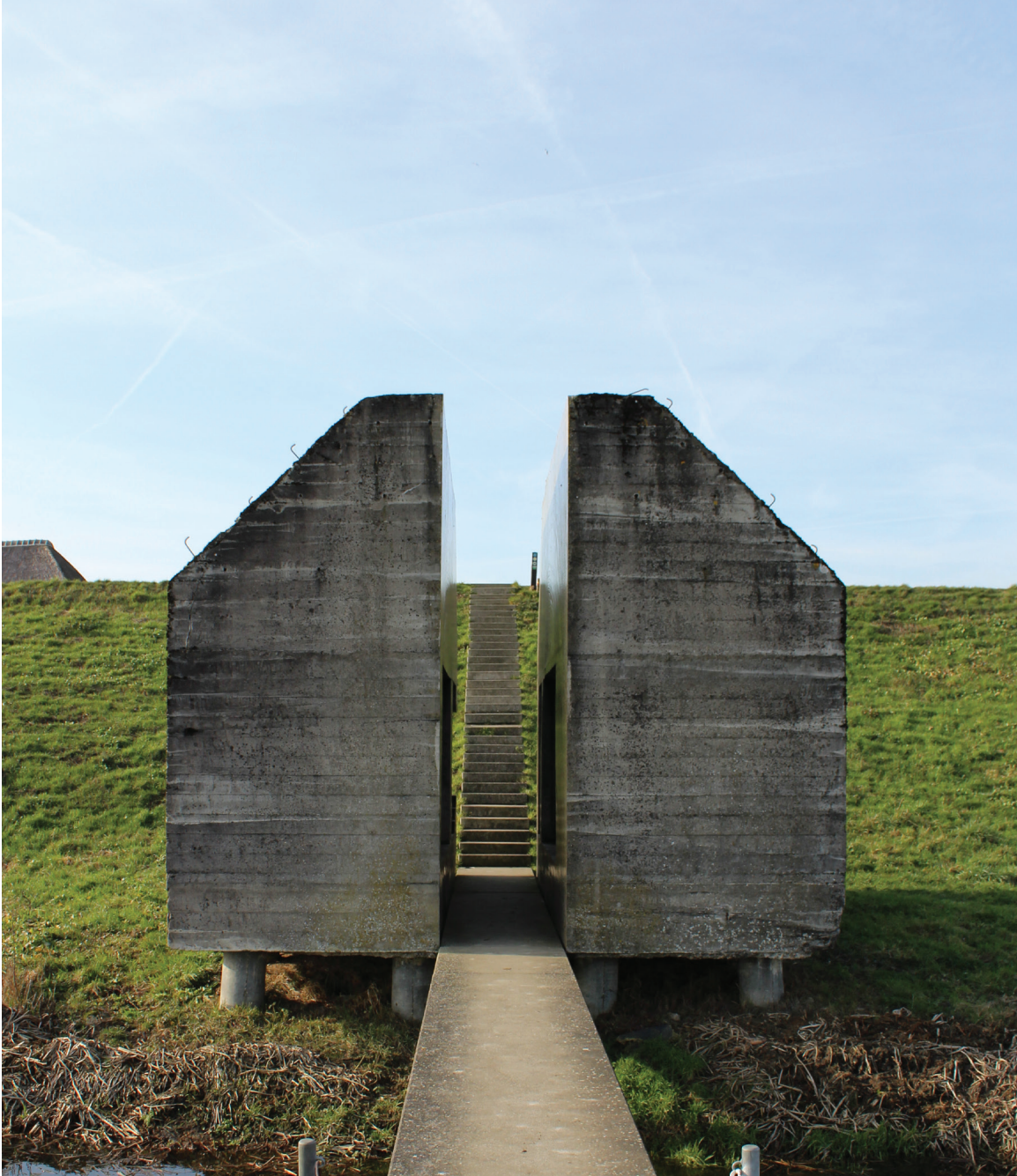
Figure 18: Bunker 599; observed February 2019
