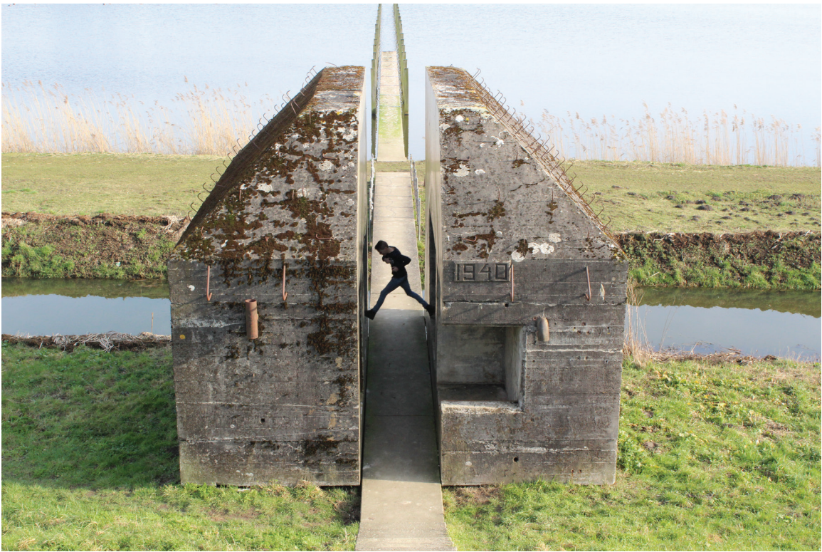
Figure 22: Bunker 599, observed February 2019
