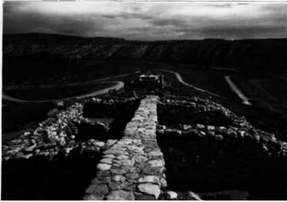
Figure 42 / Flat profile of wall caps prior to Shiner's work. Source: Shiner's 1962 Report, 33.
