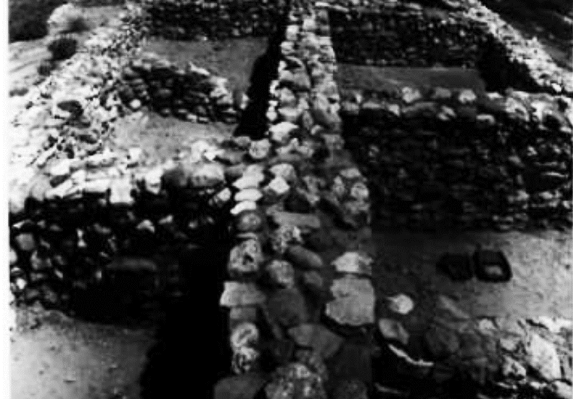
Figure 41 / New wall caps completed by Shiner. Source: Shiner's 1962 Report, 33.
