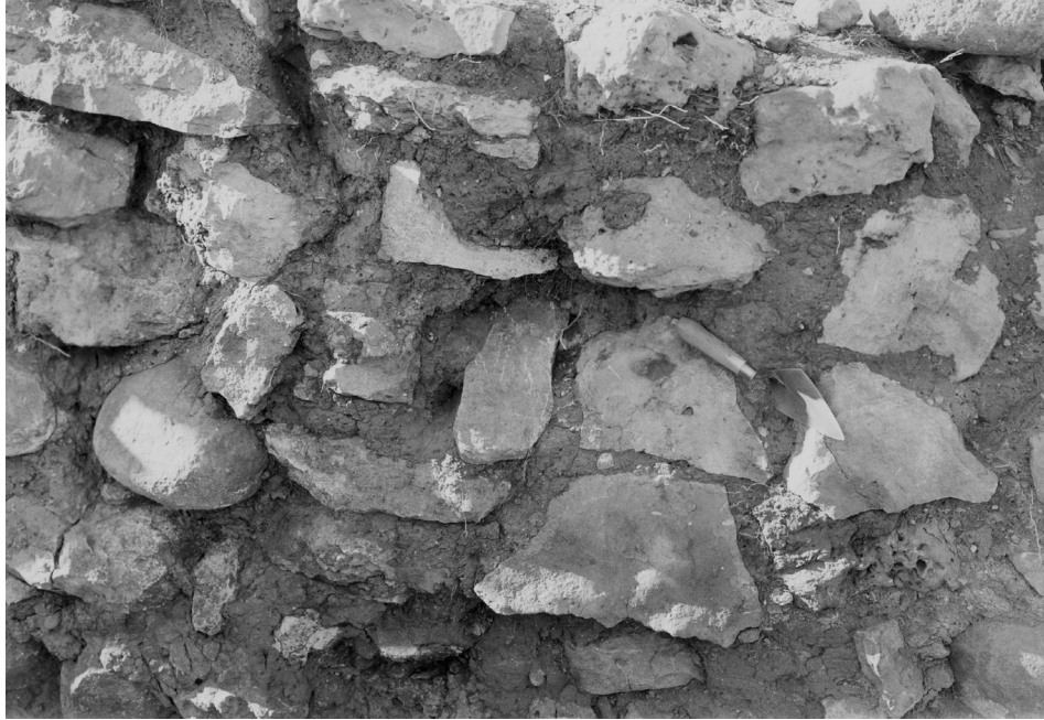
Figure 24 / Detail photo of wall as excavated. Source: Spicer and Caywood, 1933-34
