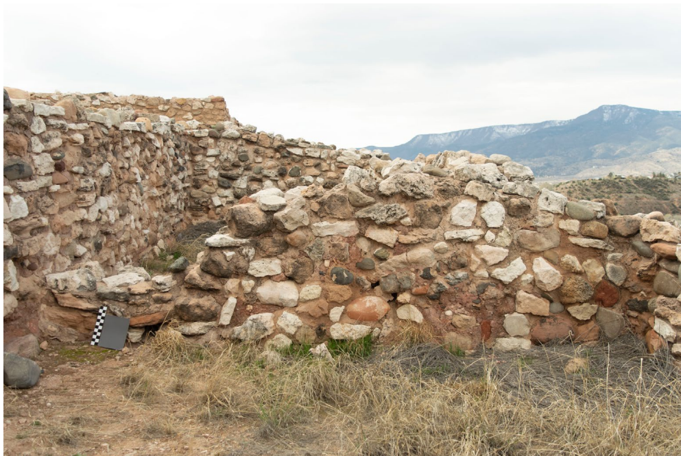
Figure 26 / Example of a wall at Tuzigoot with different mortar conditions.
