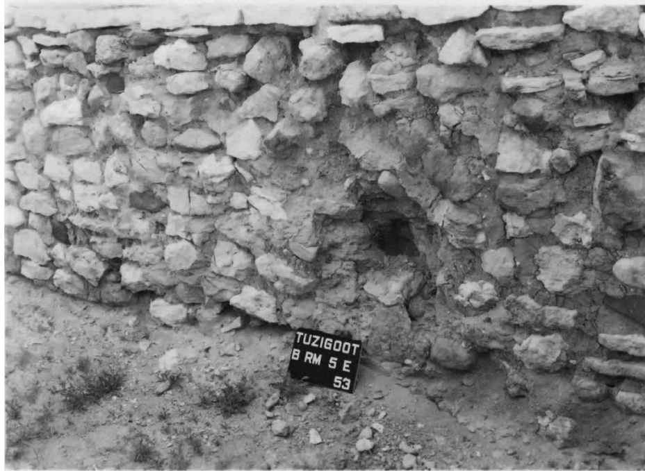
Figure 39 / Photos of damage found in wall segment 4C (east wall of room III-5) prior to stabilization completed by Richert in 1953. Source: Richert, Roland. Stabilization Report Tuzigoot National Monument. (Arizona: Southwestern National Monuments Ruins Stabilization Unit Globe, 1953), 48.
