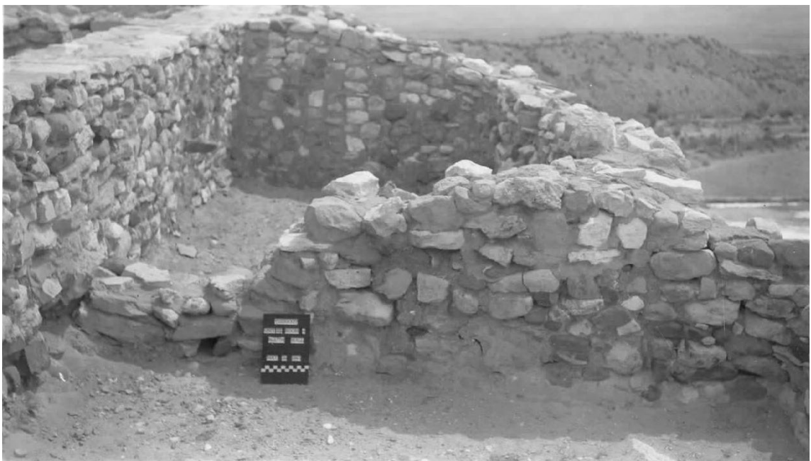
Figure 38 / Photo taken from north looking at Room III-5. Note the flat profile wall caps on the left wall (wall segment 4C). Source: 1942 Jack Cotter's photograph collection from the digital archives of Tuzigoot National Monument.
