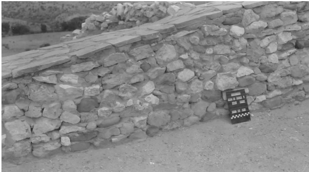
Figure 13 / Photograph showing the limestone flagstone detail of the historic visitor's trail on wall caps. Source: 1942 Jack Cotter's photograph collection from the digital archives of Tuzigoot National Monument.
