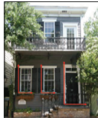
Figure 7.3: Proportionate openings along the façade.
