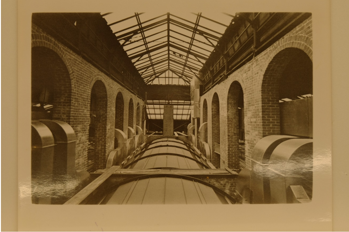
Figure 202 Detail of the skylight structure above the central hallway (Harris Davis Photography 1973)
