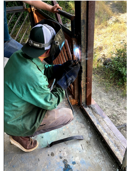
Adam Pruitt welding
