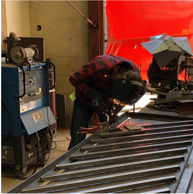
Severin Elste welding the infill
