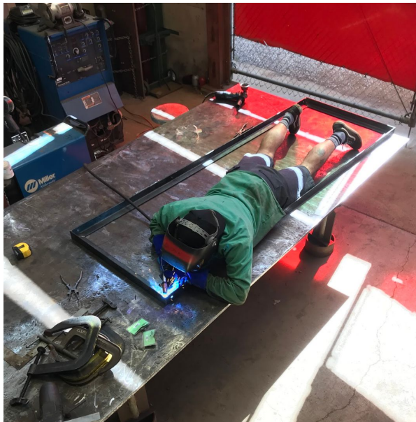
Ben Sykes welding the rectangular railing frame
