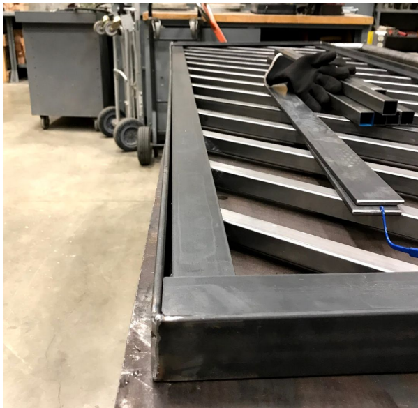
Preparing flat bar to be welded
