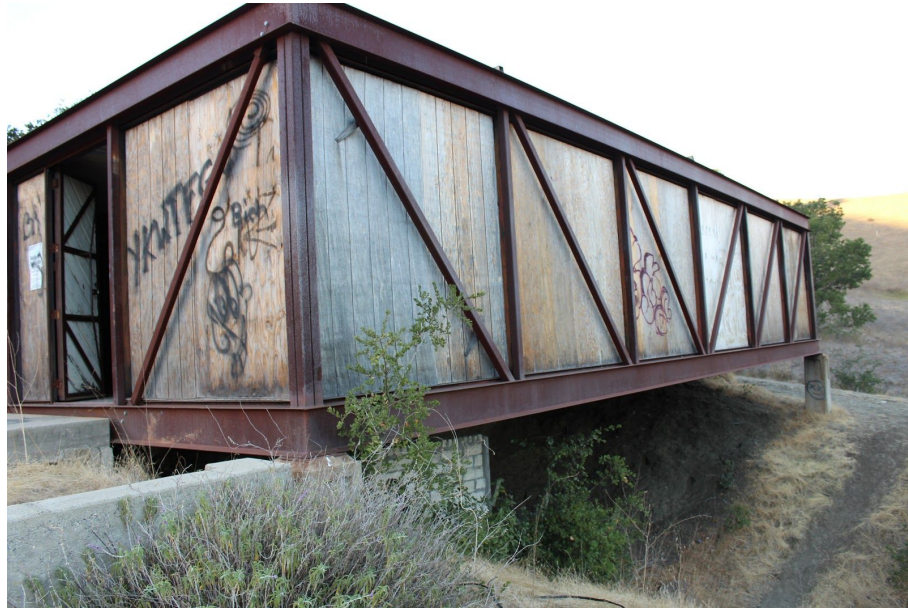
Figure 1: Bridge House in Current Condition, 2018
