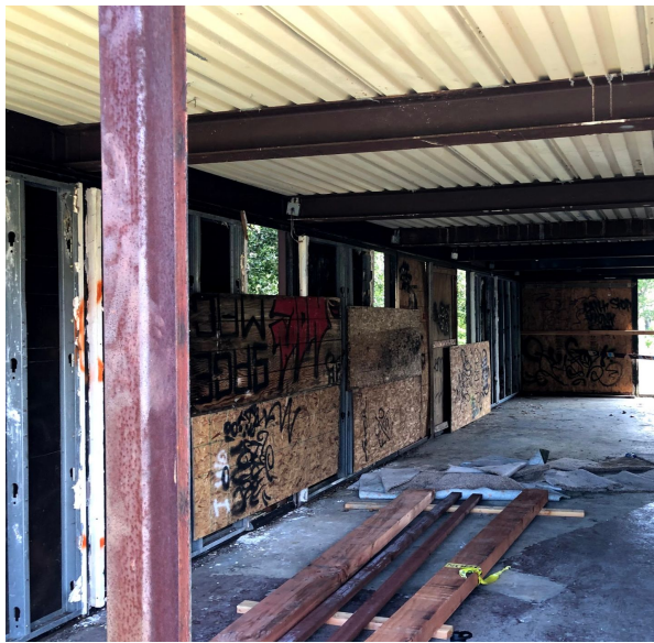
Temporary plywood barricades put in place after our first demo day
