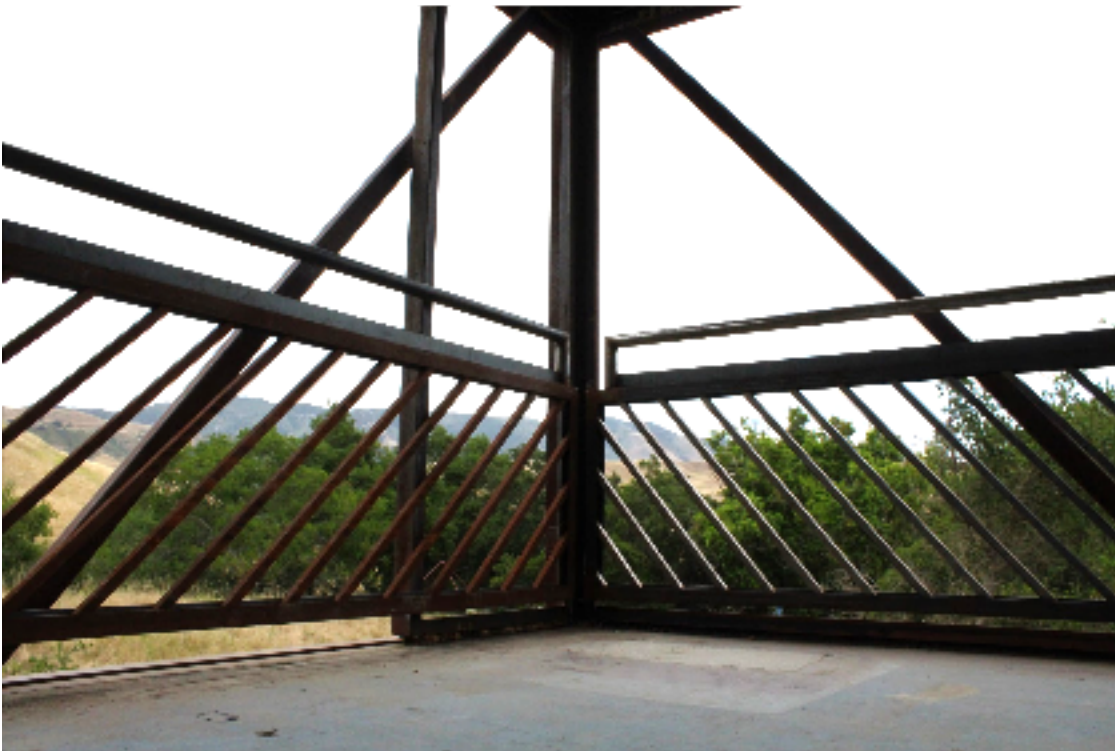
Project South-East corner
