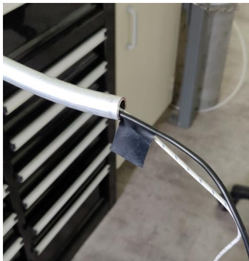
Figure 7. Stopping when the tape reaches the end of the tube
