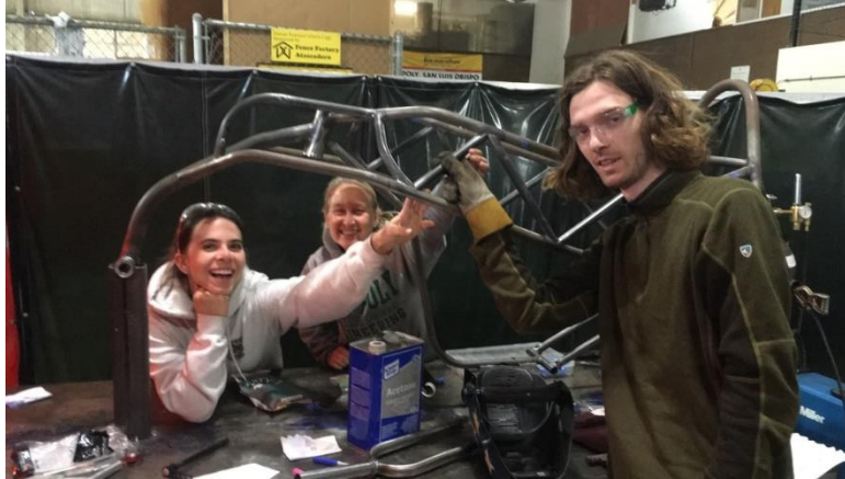
Figure 77. Eliot Briefer, Keyanna Henderson, and Kyra Schmidt, with the last truss member to go into the frame.
