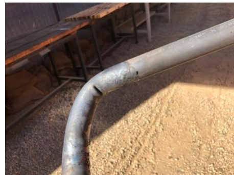
Figure 140. Bent tube showing failure by crinkling.
