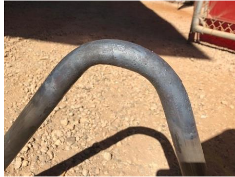
Figure 138. Bent tube showing no failure.
