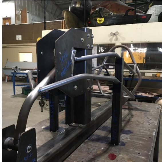
Figure 71. First stage frame jig with all members except mid-drive truss members, as built.
