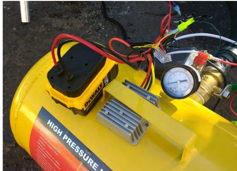
Figure 8. Battery unit connection
