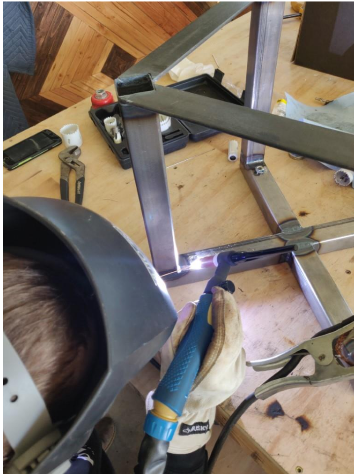
Figure 27. Welding Frame Base
