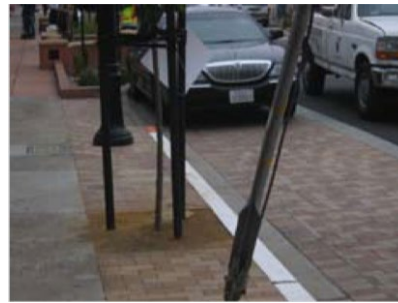
Figure 14: Pervious paving in the sidewalk and parking lane Source: Guide to the San Francisco Better Streets Plan
