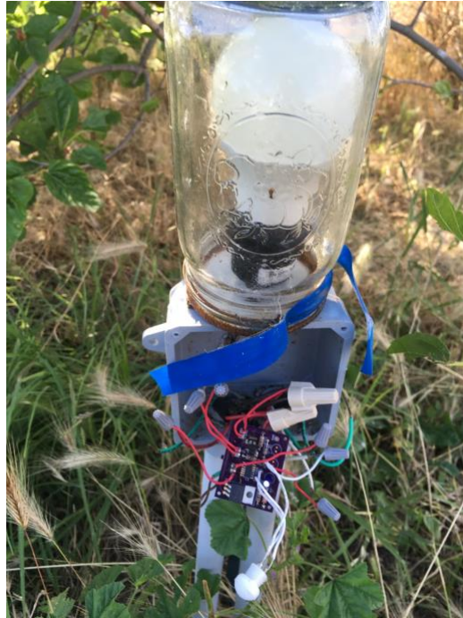
Figure 5-7: Installed circuits with LED and mason jar to protect the light bulb from weather conditions and ecosystem around the lighting pathway
