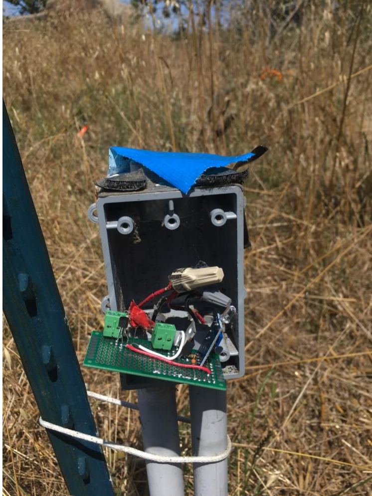
Figure 5-12: Installed ambient lighting circuit
