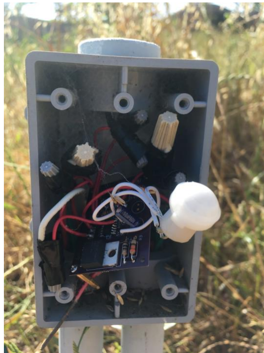
Figure 5-3: Installed circuits into circuit housing located at the DC house.
