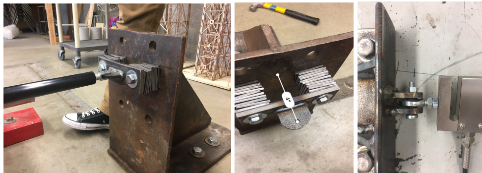
Figure 3.2.1 Detailed image of placement of pinned connection of damper to angled base plate.
