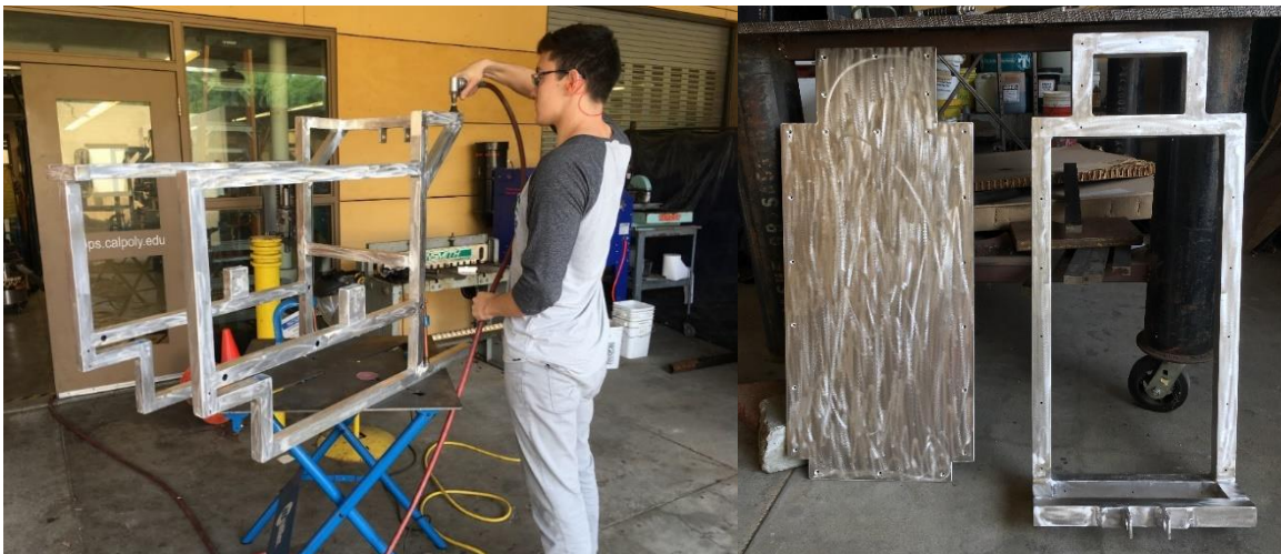
Figure 41. Completed frame and platform during paint preparation.
