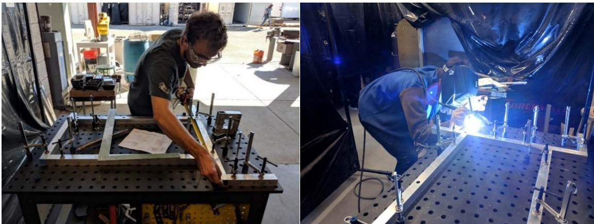
Figure 35. Jigging side of frame to welding table (left) and starting to weld (right).
