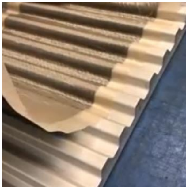
Figure 5.4. Trapezoidal shape being prepared with carbon fiber
