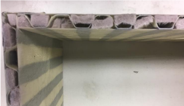
Figure 5.10. Top view of two glued walls, with aerogel installed.
