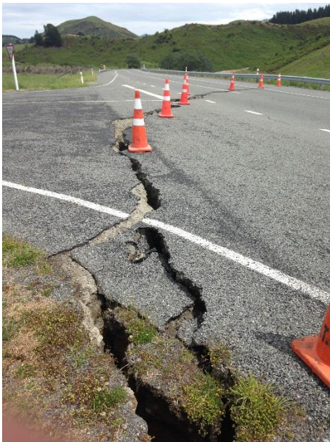
(b) Fracture Kaikoura New Zealand 2016 (reference)
