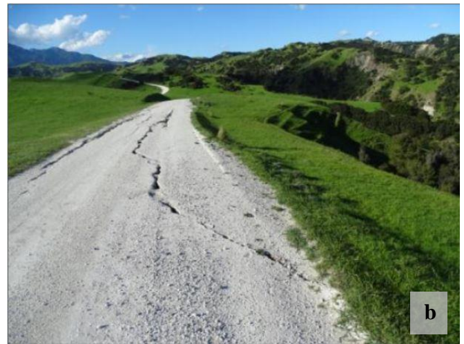
Examples of Road Fracture
